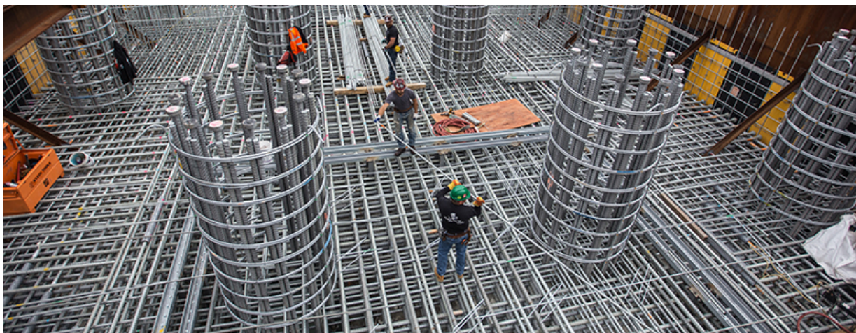
Using hot dip galvanized rebar in a structure prior to pouring concrete – galvanised rebar extends the life of bridges, waterworks structures and all manner of municipal concrete structures
