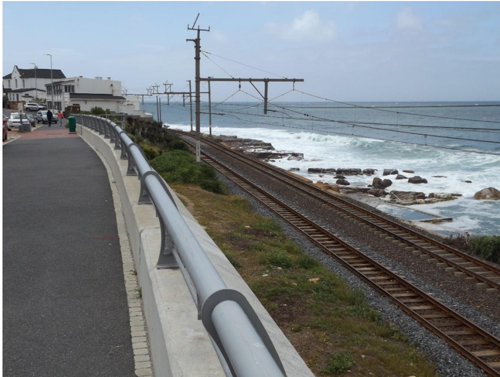
Fig 7- the new sea front retaining wall at Clovelly, Cape Town showing close proximity to the sea in False Bay & exposed to very corrosive south east wind. An ISO 9223 -C5M environment.
