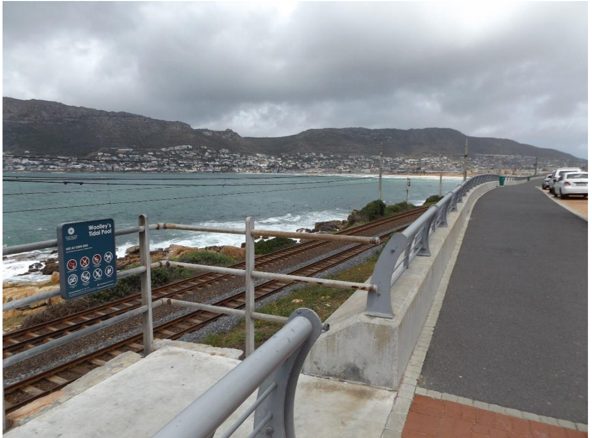
Fig 6- a new concrete sea front at Clovelly, Cape Town SA where the entire sea facing retaining concrete wall contains hot dip galvanized rebar ( author )
